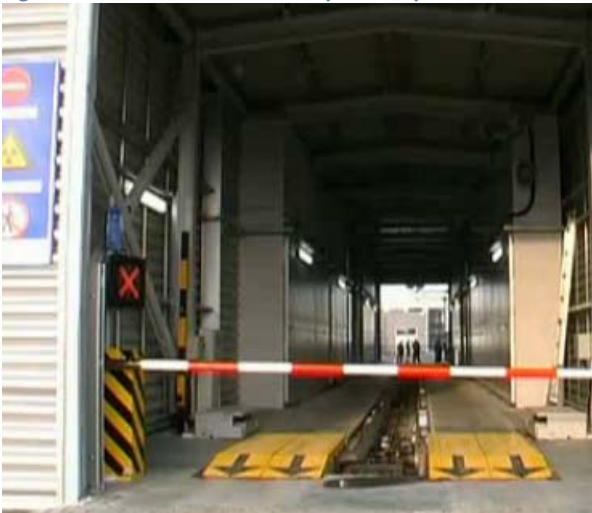
Figure 9 Container scanner in Klaipeda Seaport
